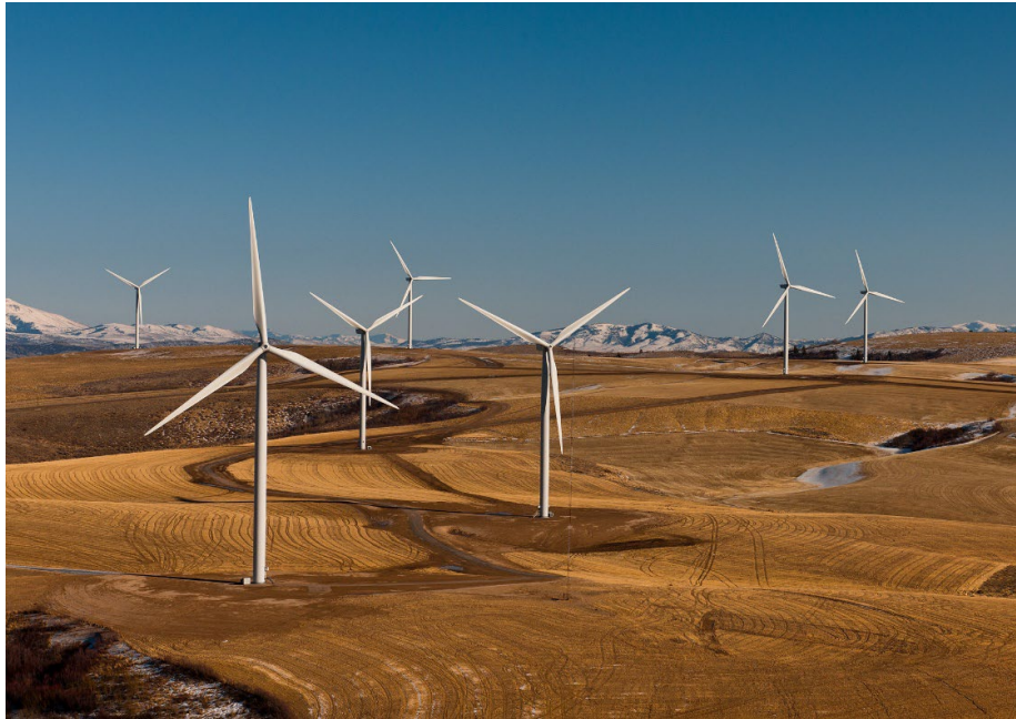
Figure 3: An aerial view of the Power County wind farm - Power County, Idaho with Nordex N100/2500 turbines. Source: U.S Department of Energy (2012).
