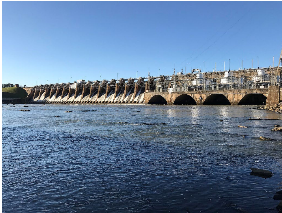
Figure 4: South side of the dam at the Tillery Hydroelectric Plant. Source: Wikimedia (2020)
