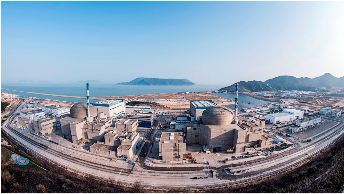
Figure 10: Taishan Nuclear Power Plant, Units 1 & 2, Guangdong, China. Source: EDF Energy (2019).
