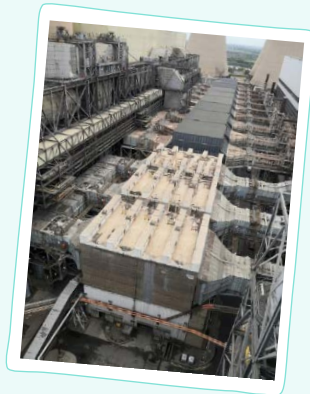
Electrostatic precipitator units at Drax - view from ground level (left) and above (right)
