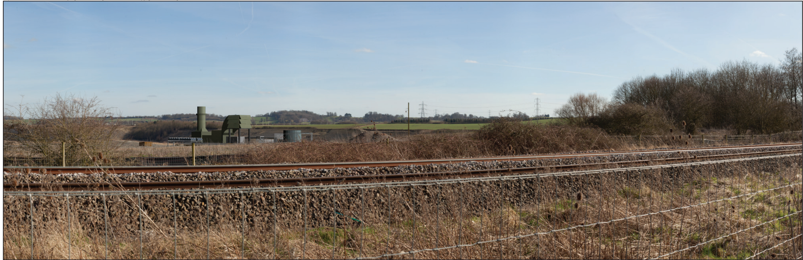
Photomontage view from Footpath within Country Park, near railway showing the Project. (72 degrees horizontal field of view, 32 cm viewing distance). View direction 103 - 175 degrees.
