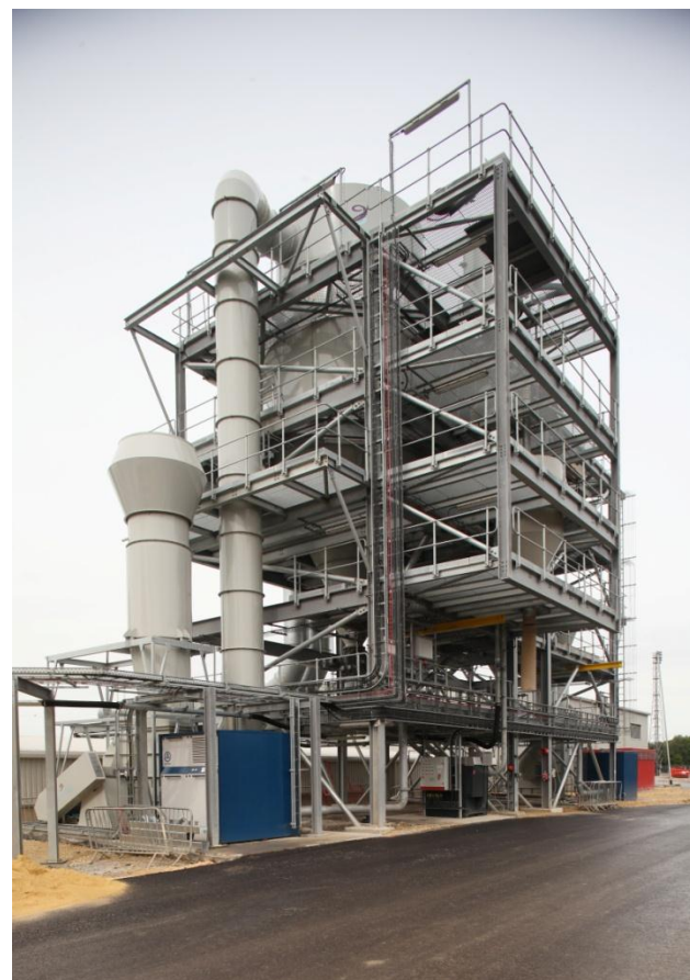
Dust Extraction System – June 2014
