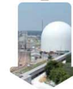
Port storage and handling
