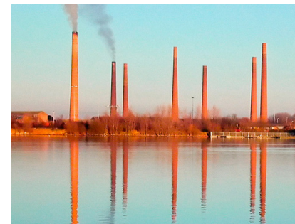
Stewartby Brick Works
