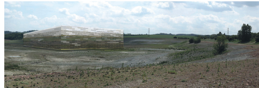
Defined horizontality on building elevation in response to horizontal landscape strata & backdrop.
