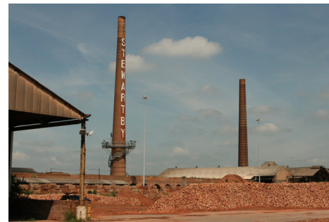
Stewartby Brick Works
