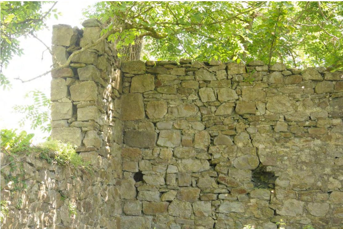
Photograph 18: Building 11 – Wall structure.
