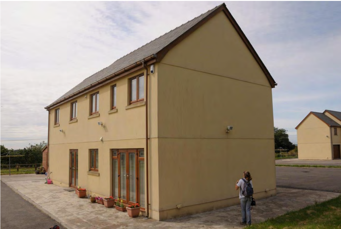
Photograph 1: Buildings 1 and 2. These houses are the same design.
