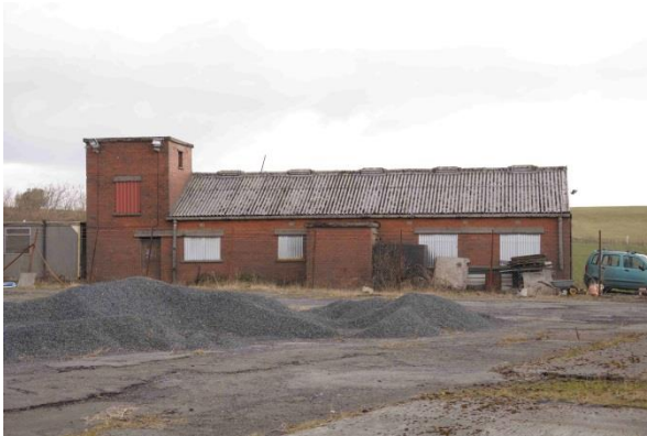
Photo 30: Building adjacent to barn at Photo 4
