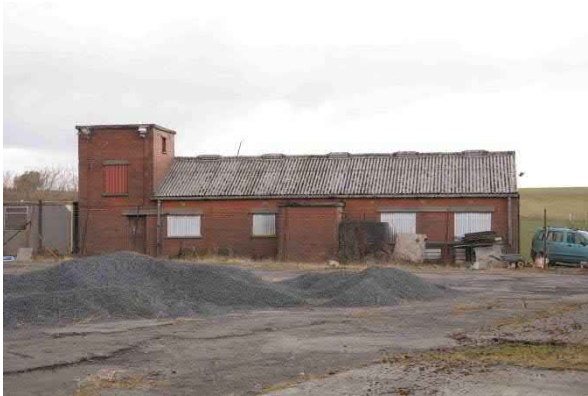
Photo 30: Building adjacent to barn at Photo 4
