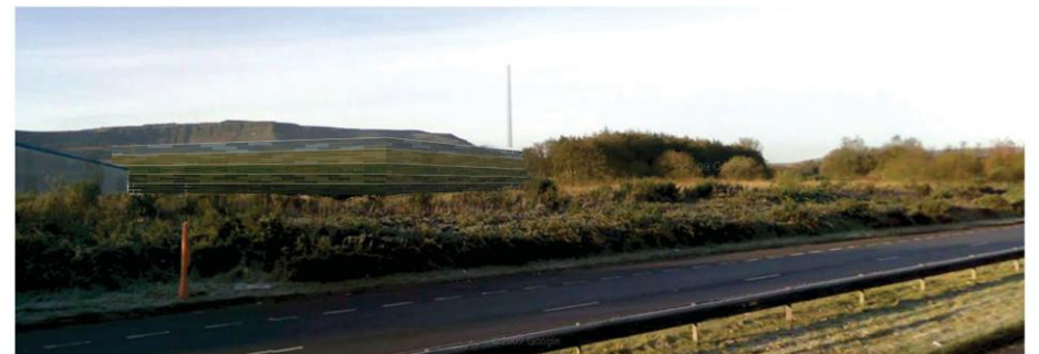
HORIZONTALITY FURTHER EMPHASIZED BY CHANNELS BETWEEN COLOUR TONES- SCALE OF THE BUILDING VISUALLY REDUCED
