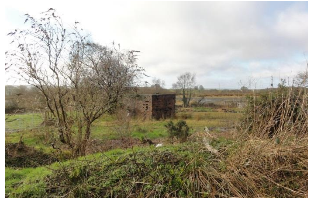
Photo 31: Bunker at TN4
