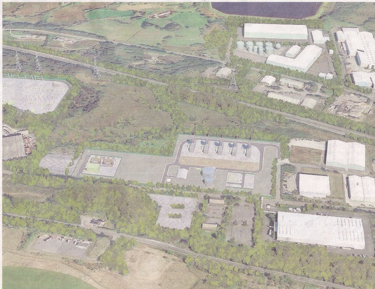
► Computer-generated image showing a proposed gas-fired power station (centre of image) at Hirwaun, proposed by Hirwaun Power. A similar scheme is now proposed north of Swansea
