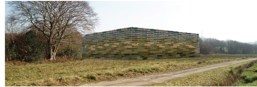
Building cladding panels arrangement as response to horizontal strata in the landscape.
